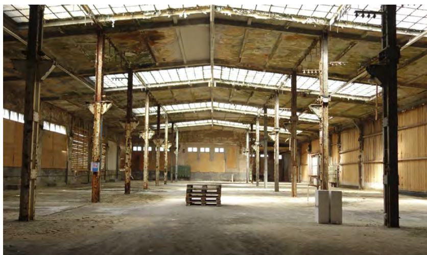
INTERIOR VIEW PITTLERWERKE LEIPZIG (2019) © PITTLERWERKE LEIPZIG, PHOTO: ANIKA DOLLMEYER
